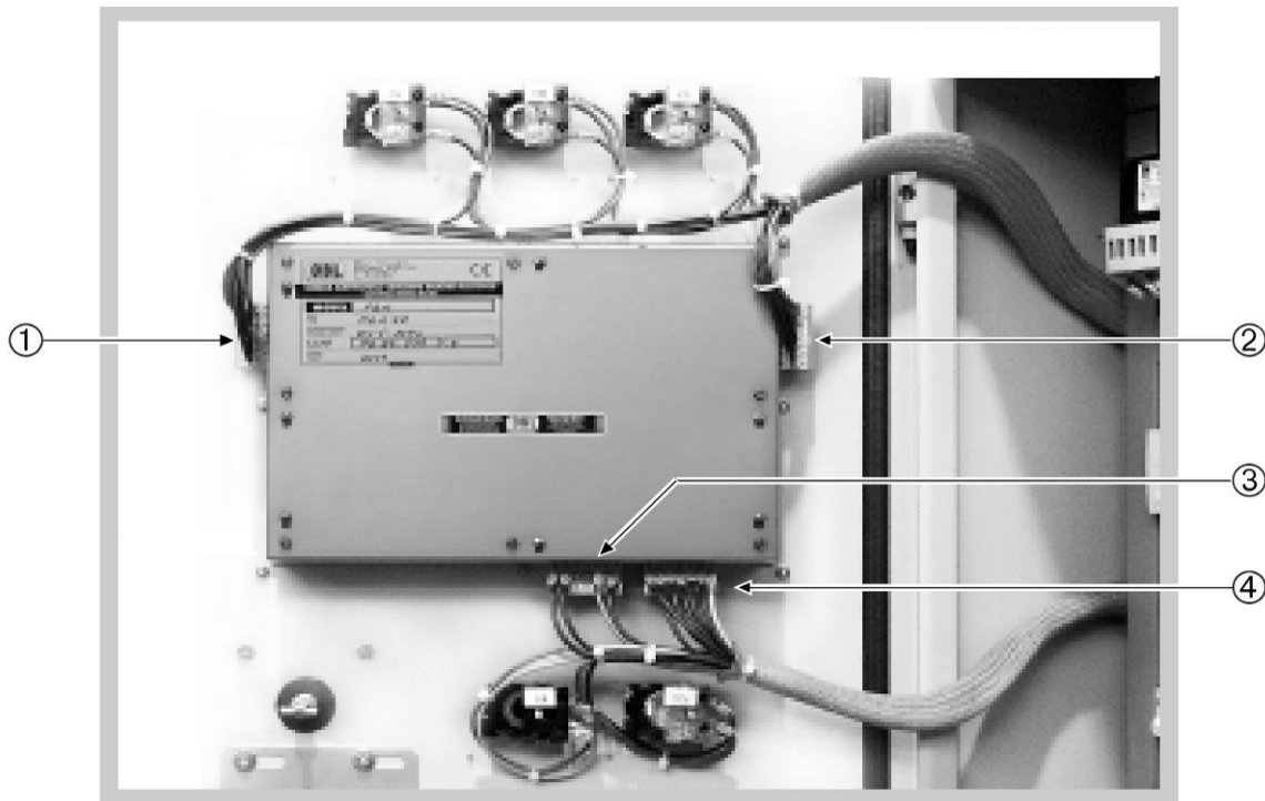
Fig. 9: Control panel replacement on electric panel
