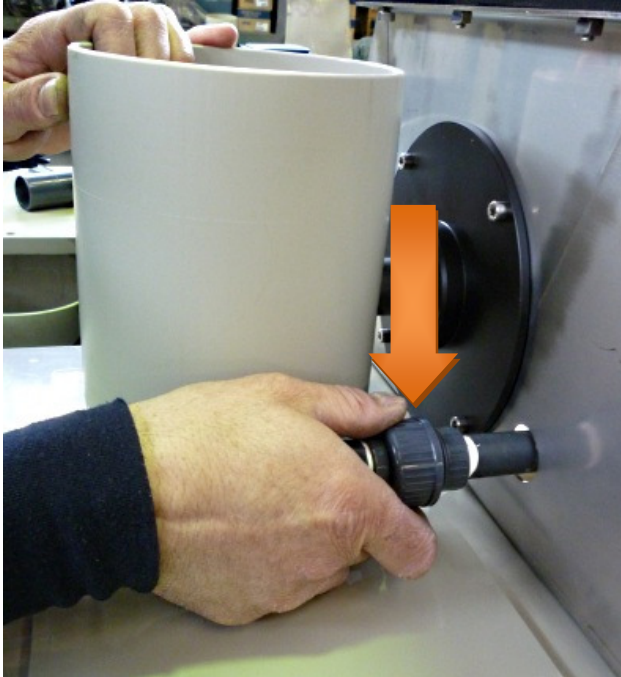
After having removed the T from inside the duct, unscrew the water supply fitting.
